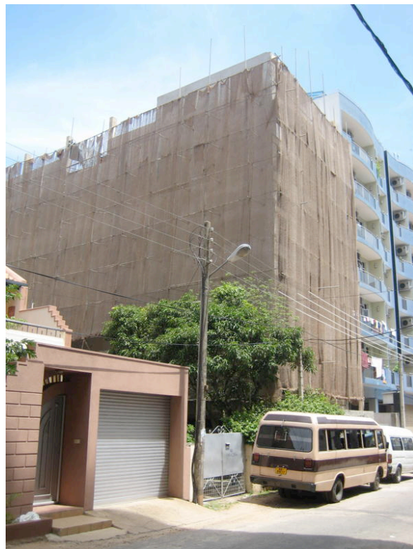
View of the progress of the KVLC construction from street view—August 2010
